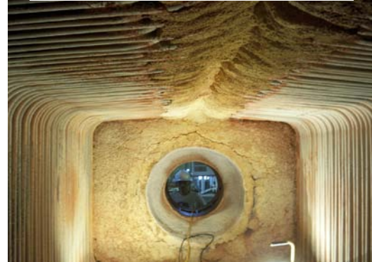
Burner Wall before application
